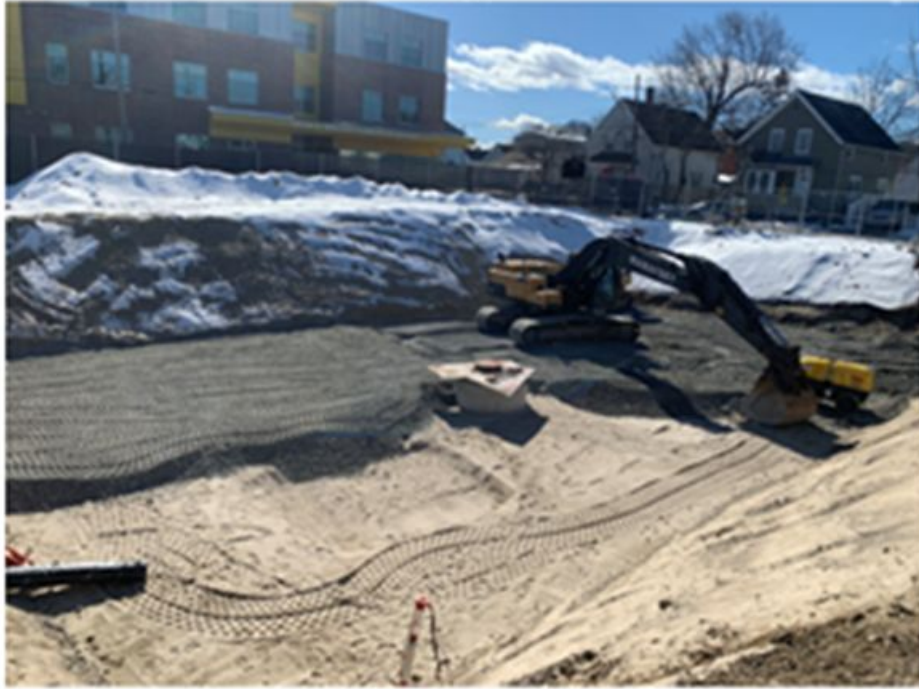
Excavation for foundations continue. Pictured above is the deep foundations for the lower-level mechanical / electrical room.
